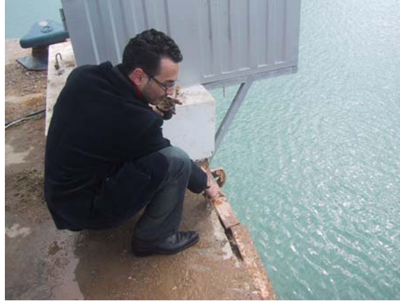
Figure 19, DPDPM Marégraphie Technician Layachi Badreddine pointing to the TGBM. Radar/microwave guide antenna just visible at base of cabinet.
