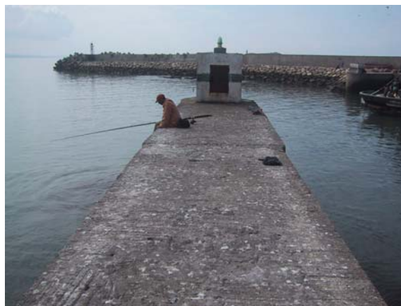
Figure 11, Essaouira Harbour entrance eastern jetty with electrical power available at the navigation light. Potential location for a radar tide gauge.
