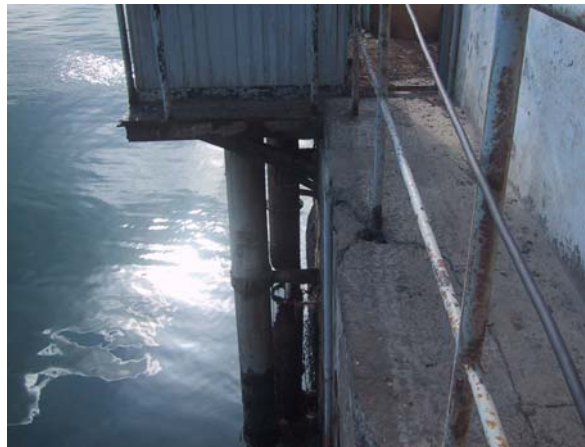
Figure 13, Old Port TG and rusting stilling wells
