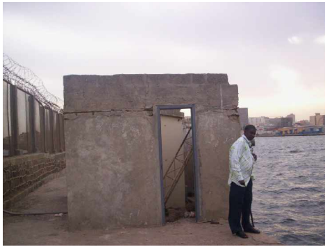
Figure 4: Old tide gauge housing at Dakar port
