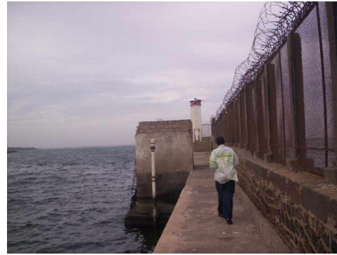
Figure 4: Old tide gauge housing at Dakar port
